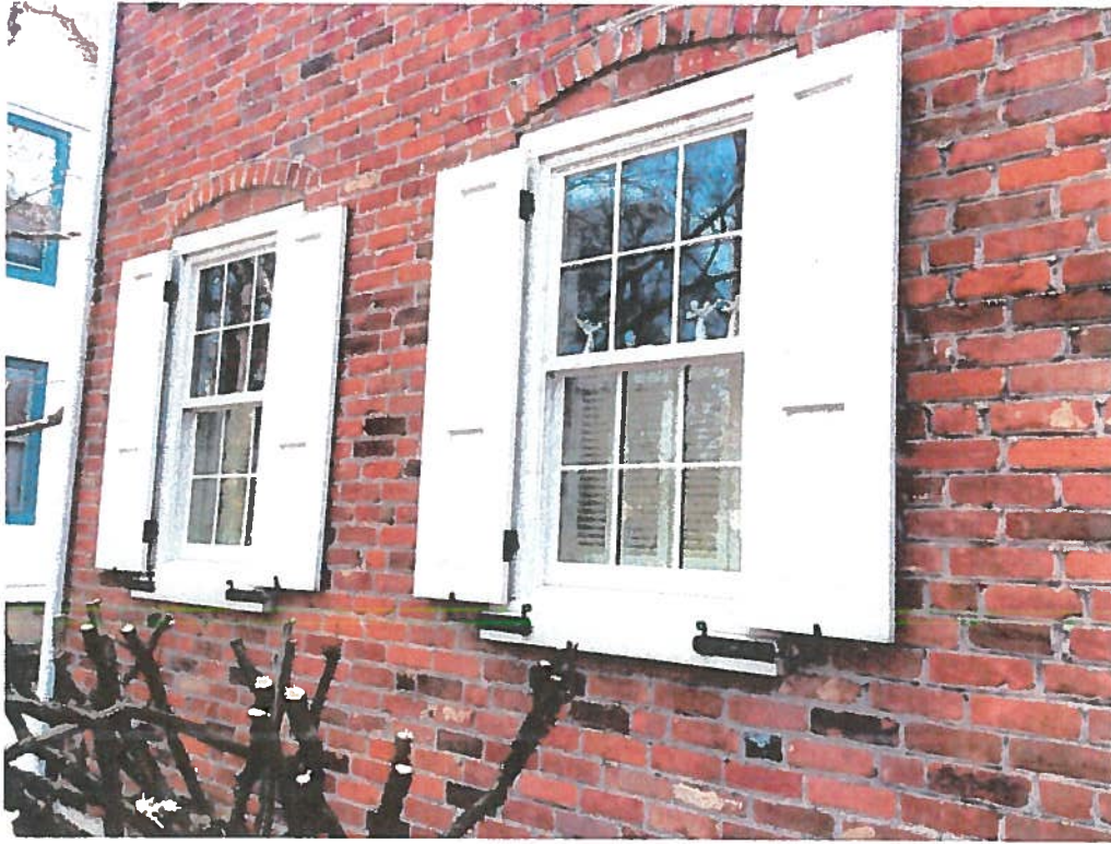
Figure 6. Anderson Woodwright Series 400 windows at 54 E Wall St – School St side of house
