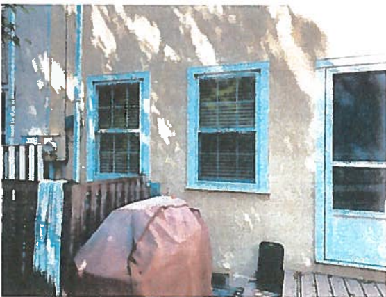
Figure 10. Two windows to be replaced with single larger window.
