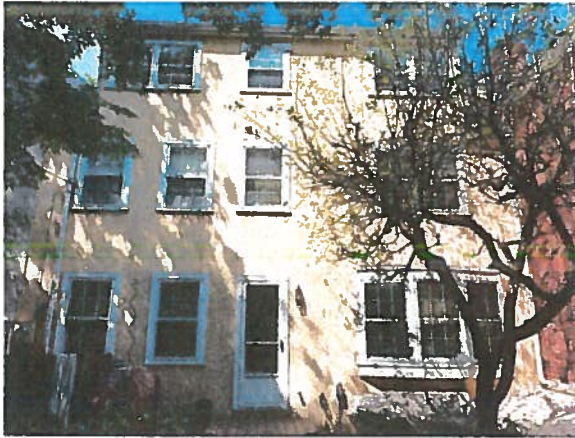
Figure 9. Rear of house
